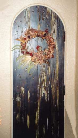
Pecky cypress was a favored material for Mediterranean Revival houses in the 1920's. Artist/builder Sam Stoltz used it frequently. Doors such as the one in the tour house at 1314 Eastin were almost a Stoltz trademark.
